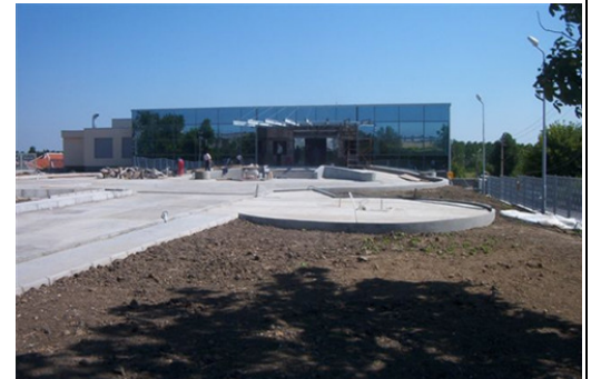
ENEMONA office Building, Kozloduj
